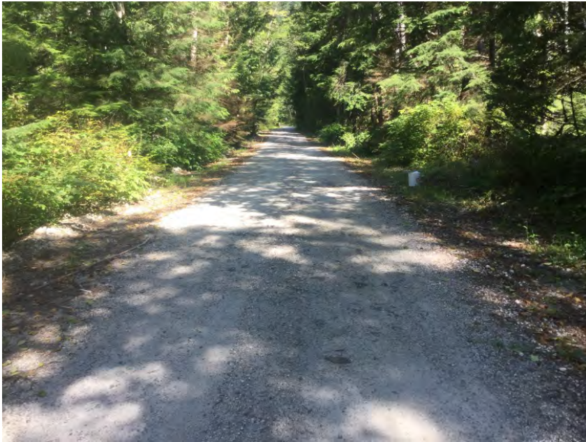
Left Approach Facing Culvert
