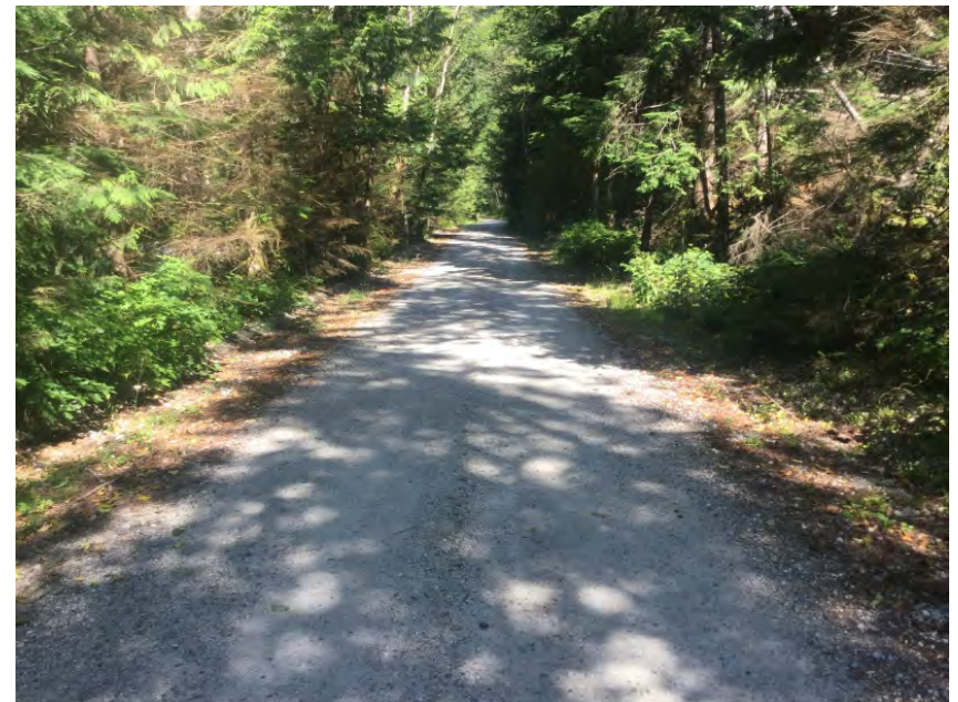
Right Approach Facing Away From Bridge
