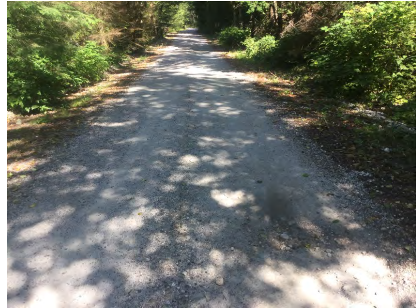
Roadway Over Culvert
